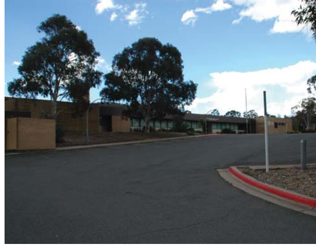
CARPARK ENTRANCE TO PRIMARY SCHOOL
