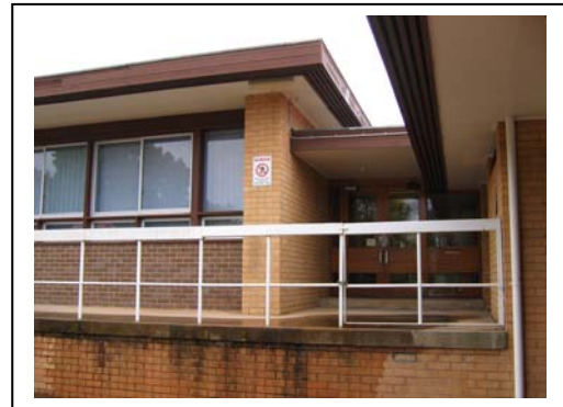
Above left and above: perimeter asbestos cement eave soffit sheet
