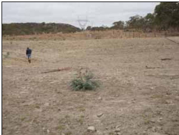
Figure 7.1 View of the transmission easement looking east from tower 134, showing constructed bank across natural creek line and associated disturbance
